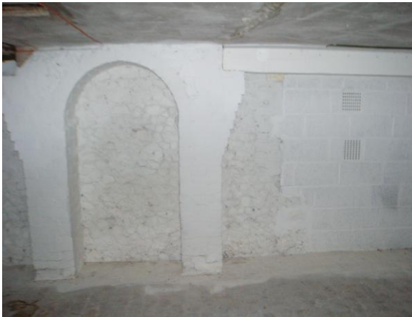
Cellar showing the building method, photo by Alix Hickman 2008
