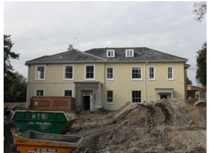
The East Elevation 2009, courtesy of Health Etcetera
